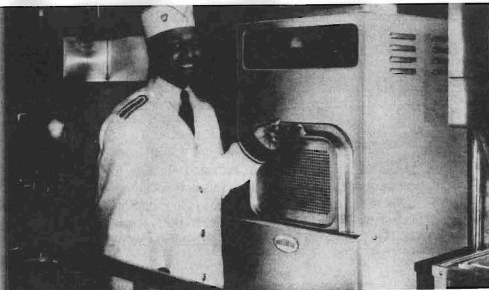
The first microwave ovens were too big for the home. Tilting the scales at 750 pounds, this one found its home on ships and trains.
