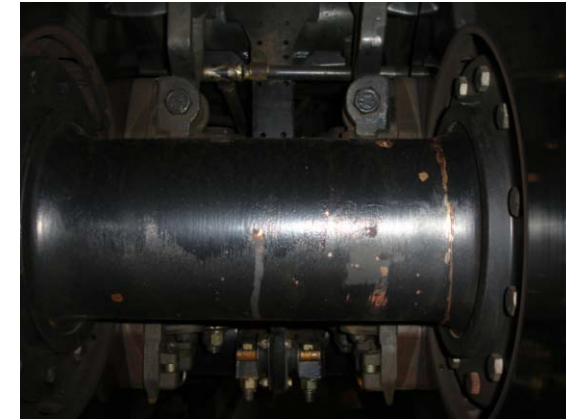
Contact with external element and starting of corrosion
